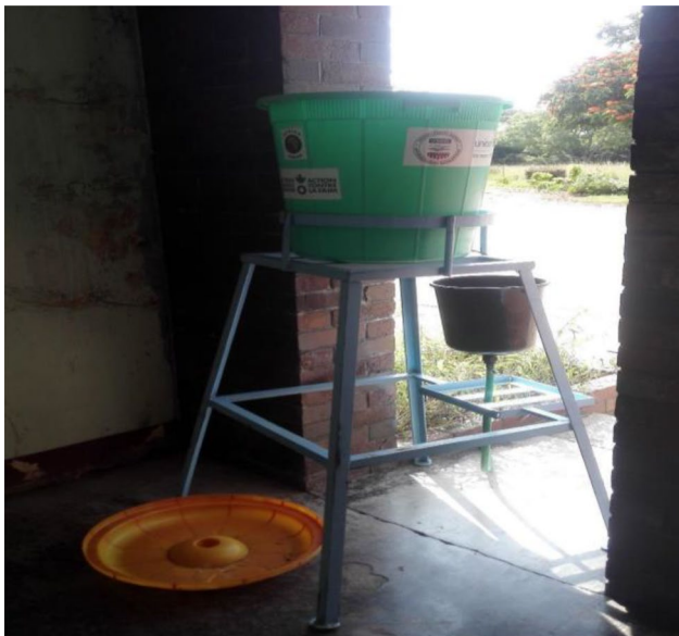
Plate 2 Washing hand facility (bucket) observed at driefontein sanatorium hospital. Source Field Survey (2023)
